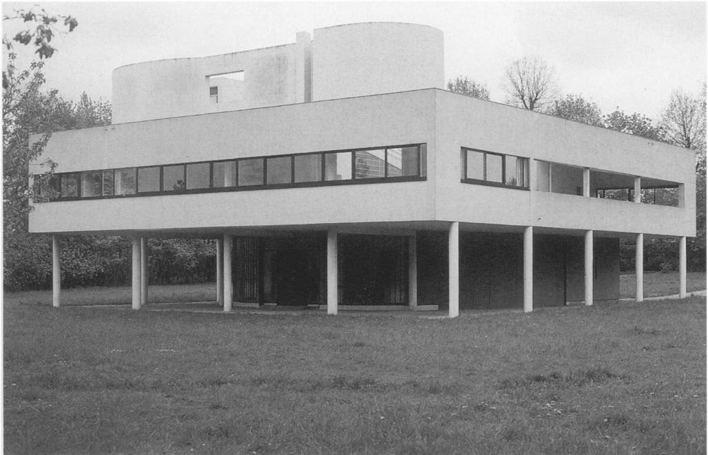
Figure 1. Villa Savoye, Poissy, was the prototype for the ‘machine for living’ set on agricultural land. It had no connection to the local environment, and even the dimensions of the villa were determined by external ones: the turning circle of the owner’s car. Photo: author.
